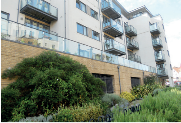
Figure 26 Screened underground parking
